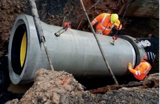
The essential advantages of Perfect Pipe have proven themselves in a multitude of projects in America, Asia and Europe: the product is corrosion-resistant, durably leakproof, easy to install and has a high static load capacity.
