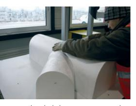
The individual cut sections are put together, the channel courses shown by a laser projection help to correctly position the moulded parts
