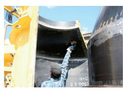
Greasing the formwork surfaces with Ortolan SEP 791 release paste from MC Bauchemie
