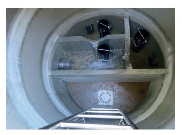
View inside a DN1500 concrete water chamber tailor-made by Wyss AG, with multiple inlets and 4 chambers at the water catchment site in the municipality of Vitznau, on Lake Lucerne.
