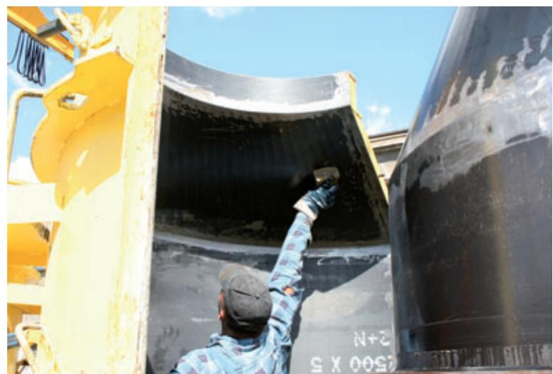
Greasing the formwork surfaces with Ortolan SEP 791 release paste from MC Bauchemie
