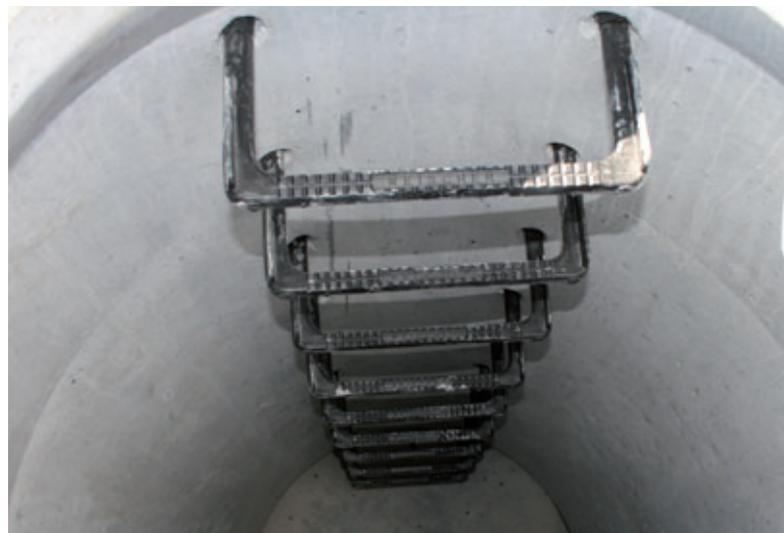
*After de-moulding, the steps are knocked into in designated bushings*
