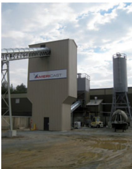
Americast's Ashland facility, which uses the Schlüsselbauer Exact 1500, has four 60-ton [55 Mg] aggregate bins, and two silos, one for cement and one for fly ash (25% of fly ash replacement for cement is permissible in the concrete mixture).
