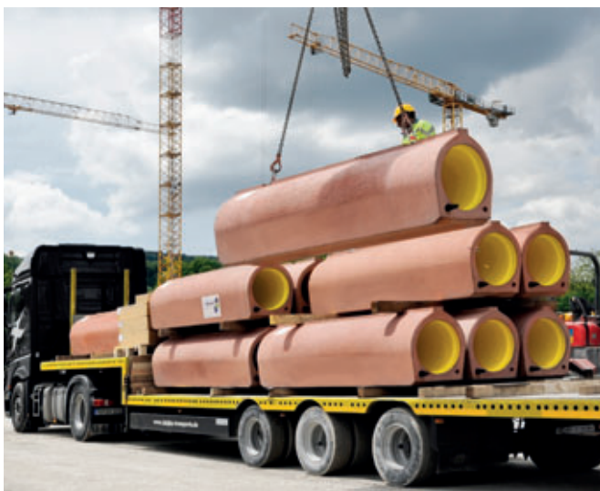
The anchors cast firmly in concrete ensure safe handling of the robust concrete pipes, with or without liner
