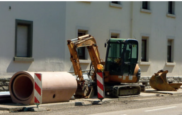
As a basis for an adjacent redevelopment, DN800 prebed concrete pipes were produced in Achern, Baden-Württemberg, some with pre-made connections for side branches on the same invert
