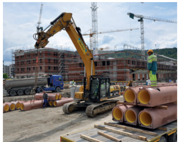
The anchors cast firmly in concrete ensure safe handling of the robust concrete pipes, with or without liner
