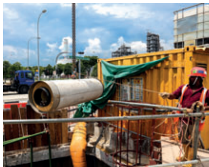
The advantages of concrete pipes – high structural load-bearing capacity and robustness for day to day work on the construction site – are intensified still further by a pipe wall thickness of 130 mm.
