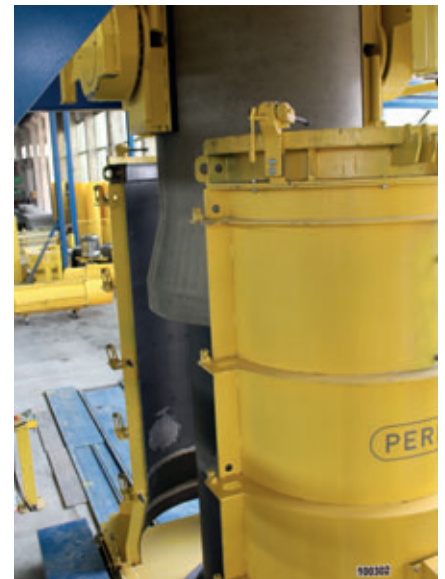
After hardening in the mould, the concrete pipes are demoulded and the connectors are mounted at each pipe end.
