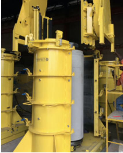
Demoulding of a cured jacking pipe
