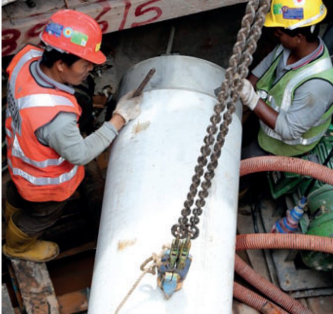
Inserting a pipe into the starting pit
