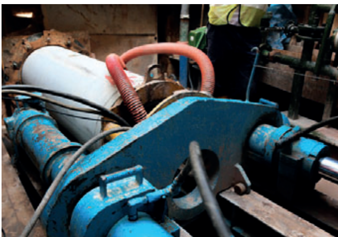
Reliable jacking of the pipe
