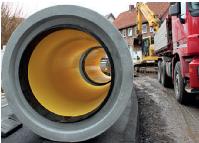
Temporary storage of DN1000 Perfect Pipe reinforced concrete pipes with pre-installed connectors at the building site in Sandershausen, municipality of Niestetal.
